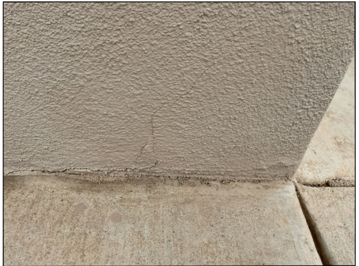
Typical Cracking of stucco, needs repairs
